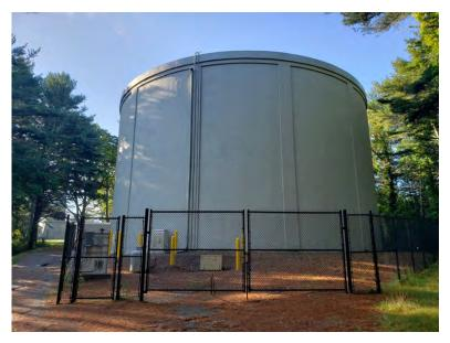
The interior and exterior surfaces were cleaned, inspected and rehabilitated at the Captains Hill Tank (*picture*). A mixing system and perimeter fencing were installed. New access hatches, vent finial and fall suppression systems were installed on the roof of the tank. The field surveying, wetland flagging, permitting and design work was completed for the 5 streets remaining with PCE water mains.
