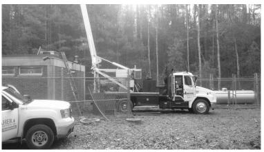
Tremont Street well site being cleaned and redeveloped to correct lost pumping capacity
