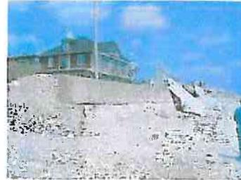
Primary Type: **Bulkhead/ Seawall** Primary Material: **Concrete** Primary Height: **5 to 10 Feet**
