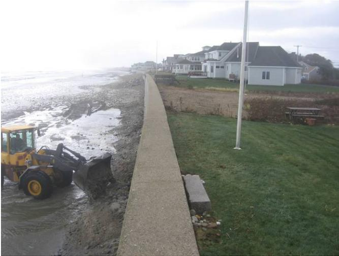
PHOTOGRAPH 29 - BACK LOADER FILLING IN FRONT OF WALL AT UNDERMINING
