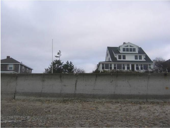
PHOTOGRAPH 21 - CHANGE IN WALL CONSTRUCTION APPROX. STA 127+00.
