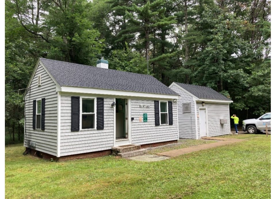
PARTRIDGE ROAD WELL PUMP STATION
