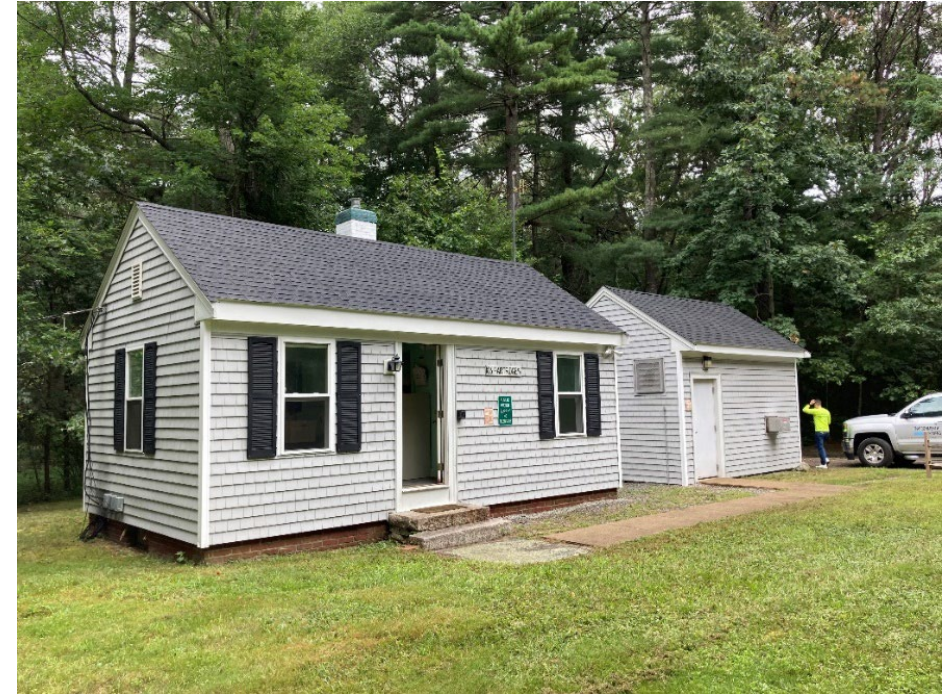
PARTRIDGE ROAD WELL PUMP STATION
