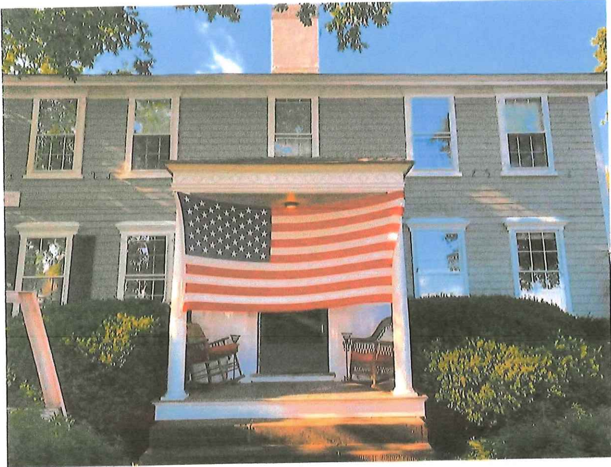
Front of house, facing south
