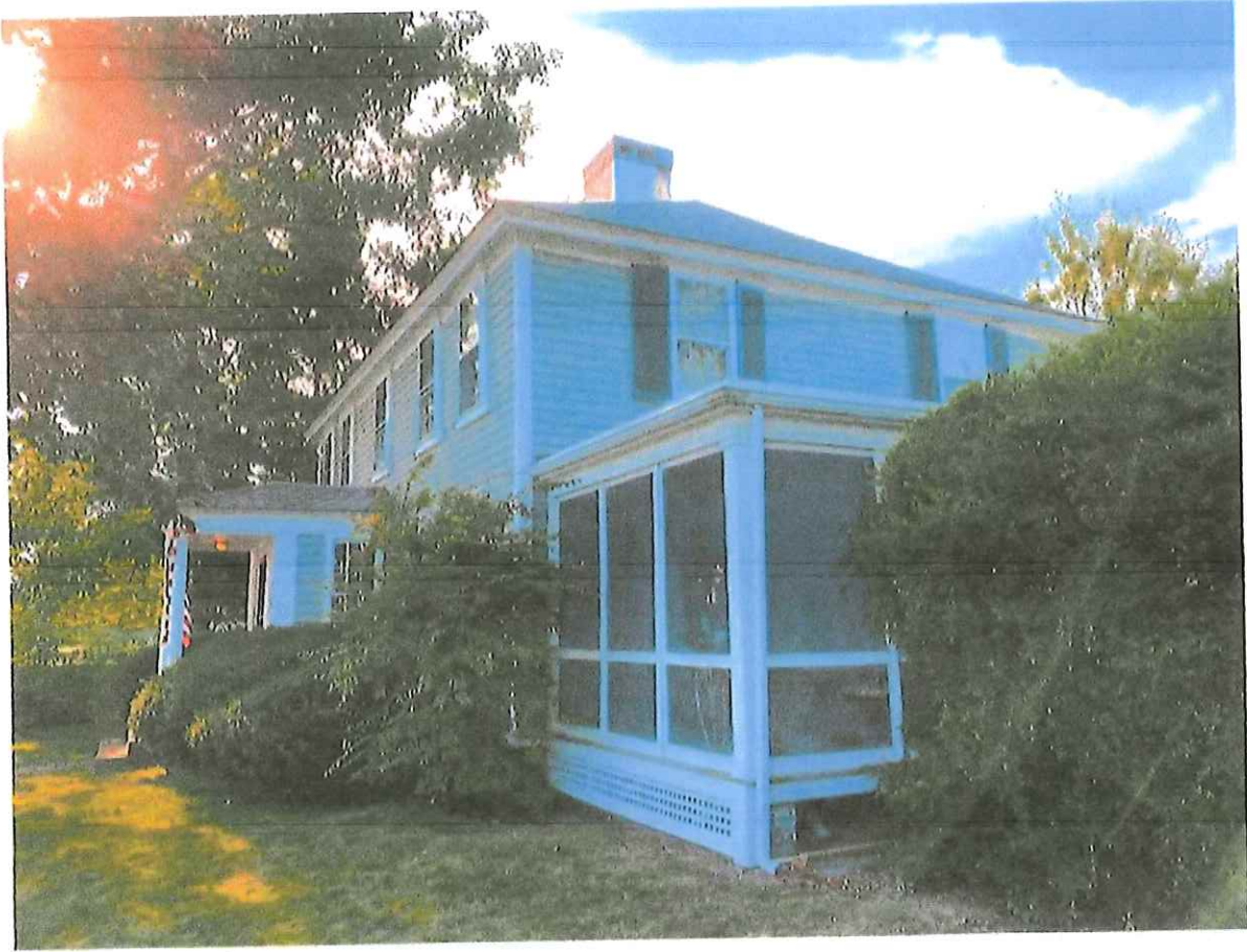
Southeast corner of house with 20 th -century screened porch.
