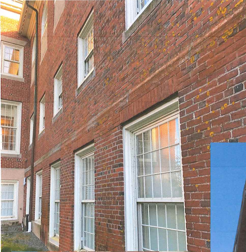
Left: detail of brick water table
