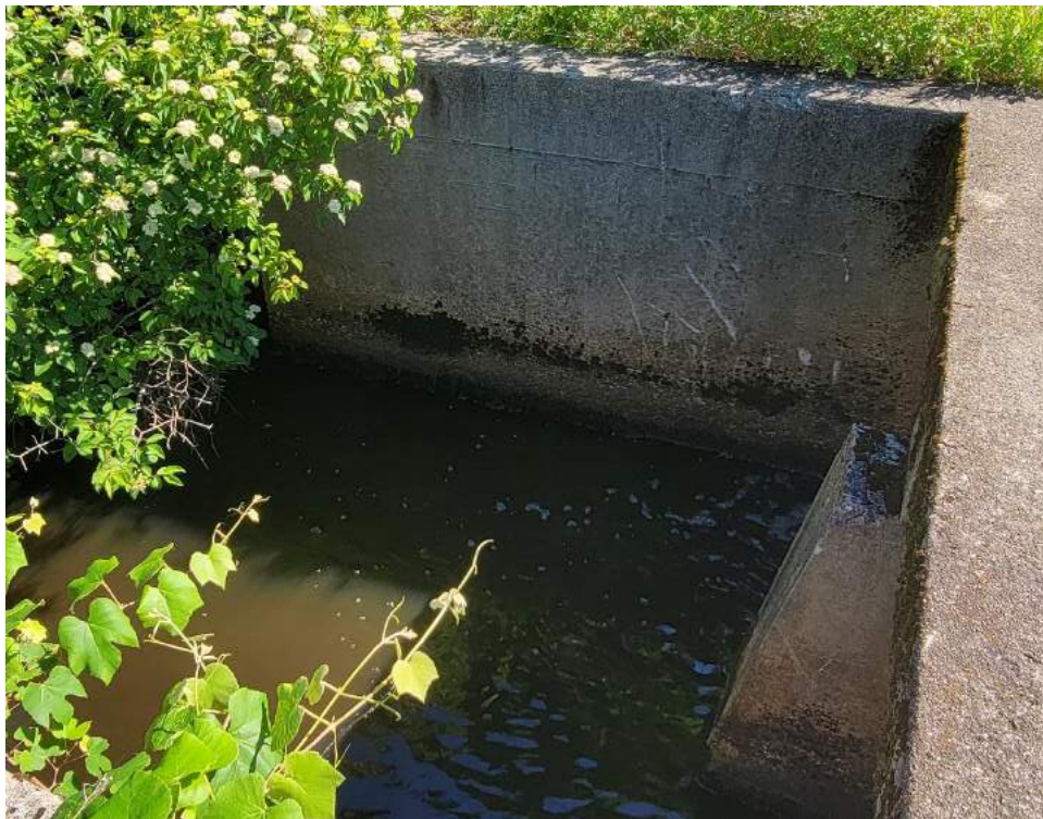
Photo 8: Temple Street Concrete Training Walls (note pier in the middle)
