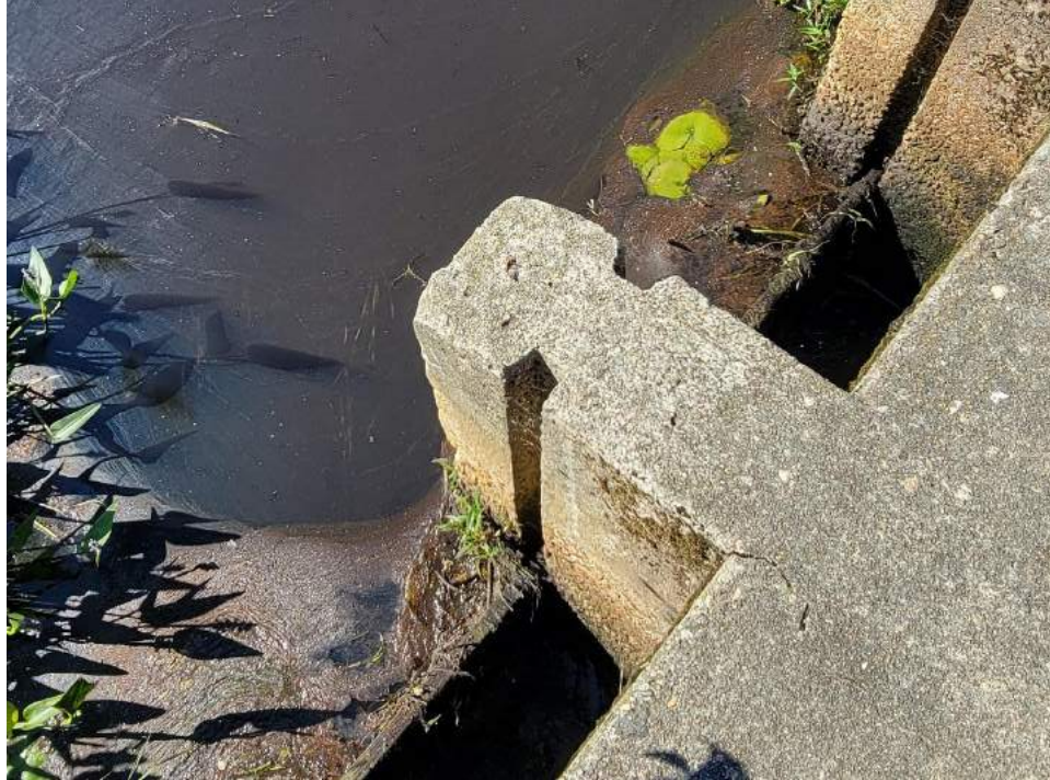
Photo 7: Temple Street Dam Outlet Structure Dagger Boards
