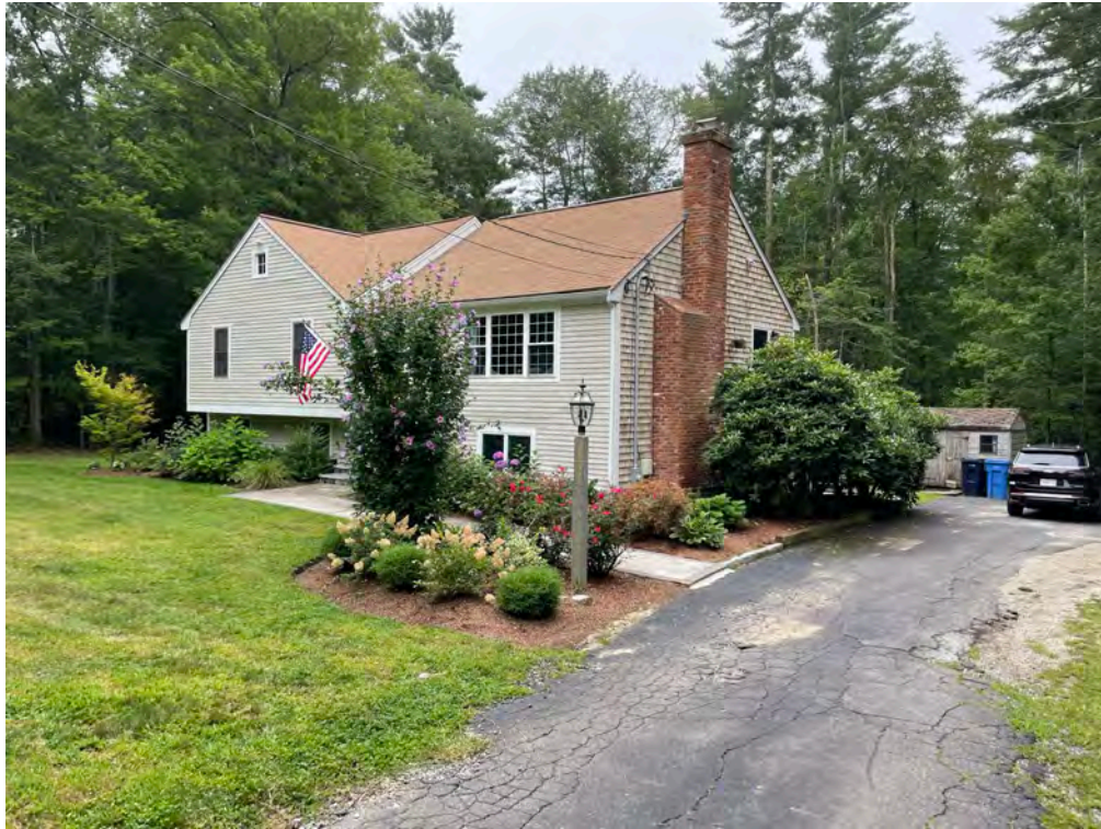
Photograph #1 – View of front of the house and location of the proposed garage & mudroom addition.
