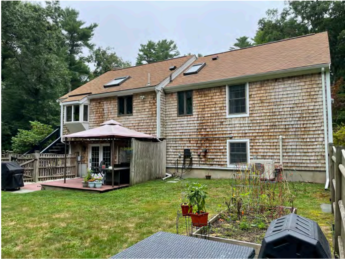
Photograph #3 – View of the rear of the house.
