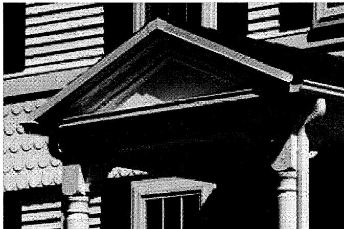
Detail of entrance on west (façade) elevation (view NE)
