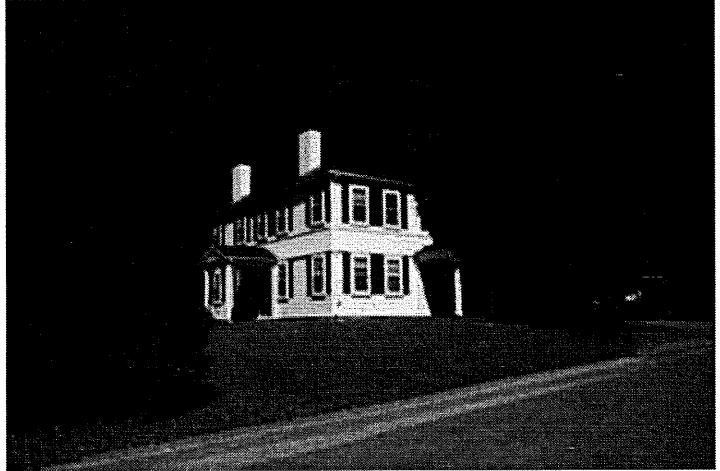
West and south facade elevations (view NE)
