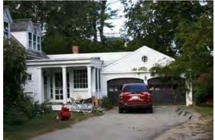
Appendages and garage: South (façade) elevation (view N)
