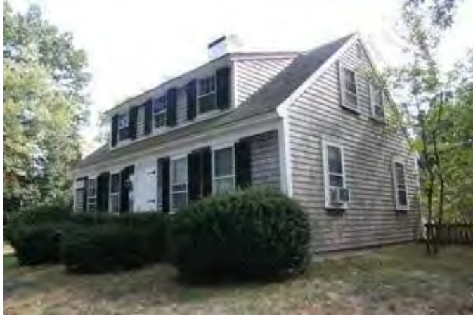
North (façade) and west elevations (view SE)
