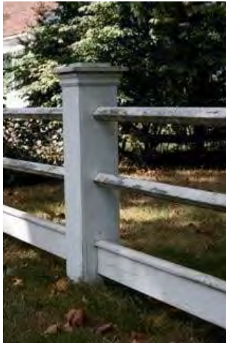
Fence detail (view NW)
