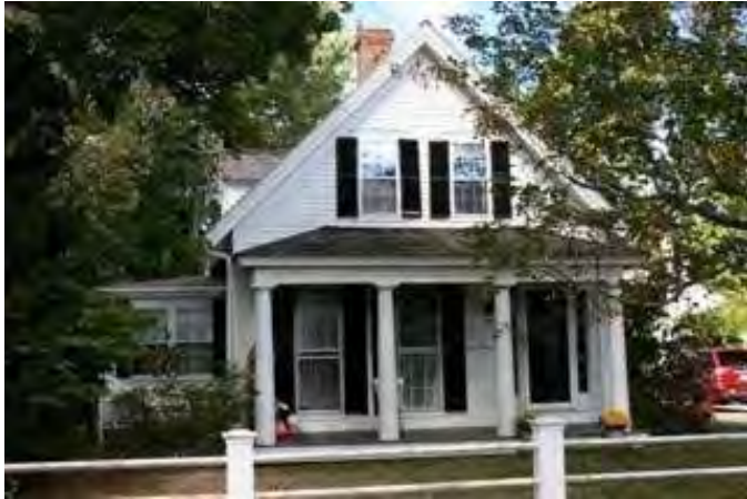
South (façade) elevation (view N)
