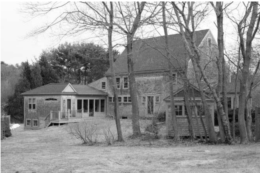
View from southwest; rear additions, barn, and free-standing shed.
