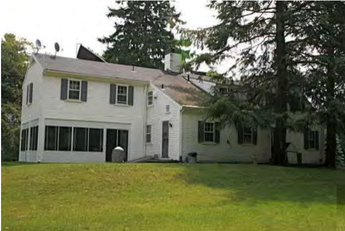
North (rear) and west (side) elevations; main block at right
