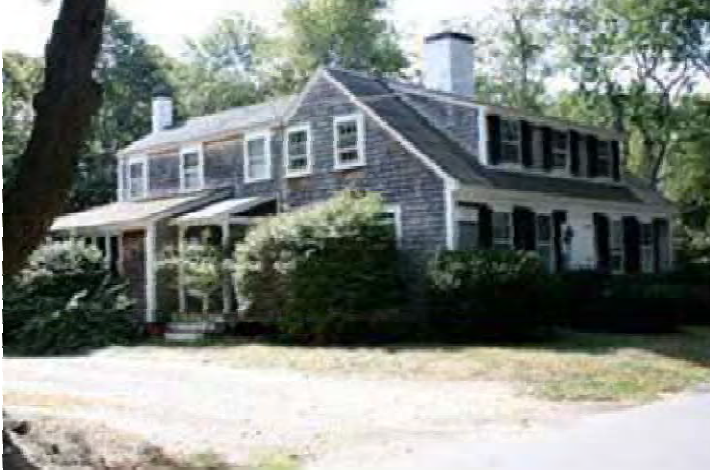
East and north (façade) elevations (viewNW)
