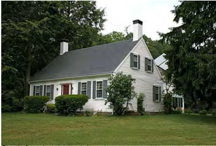
South façade and east elevation
