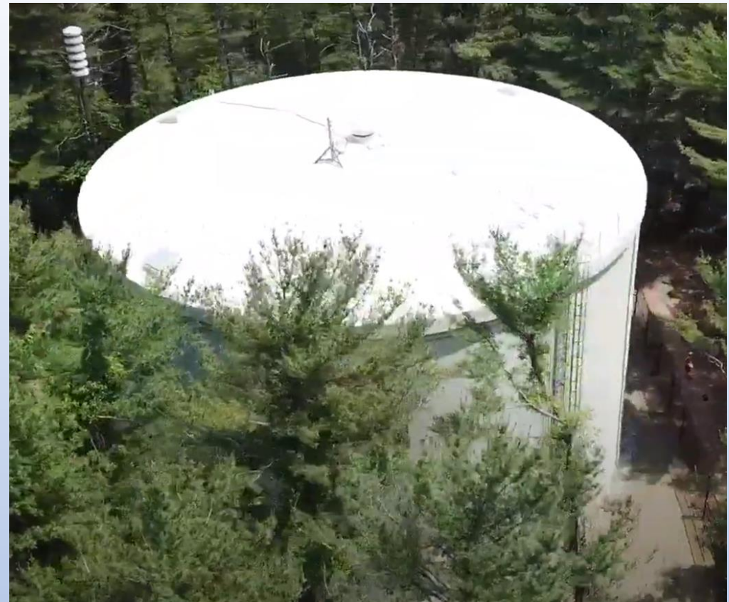
Captain's Hill Water Tank
