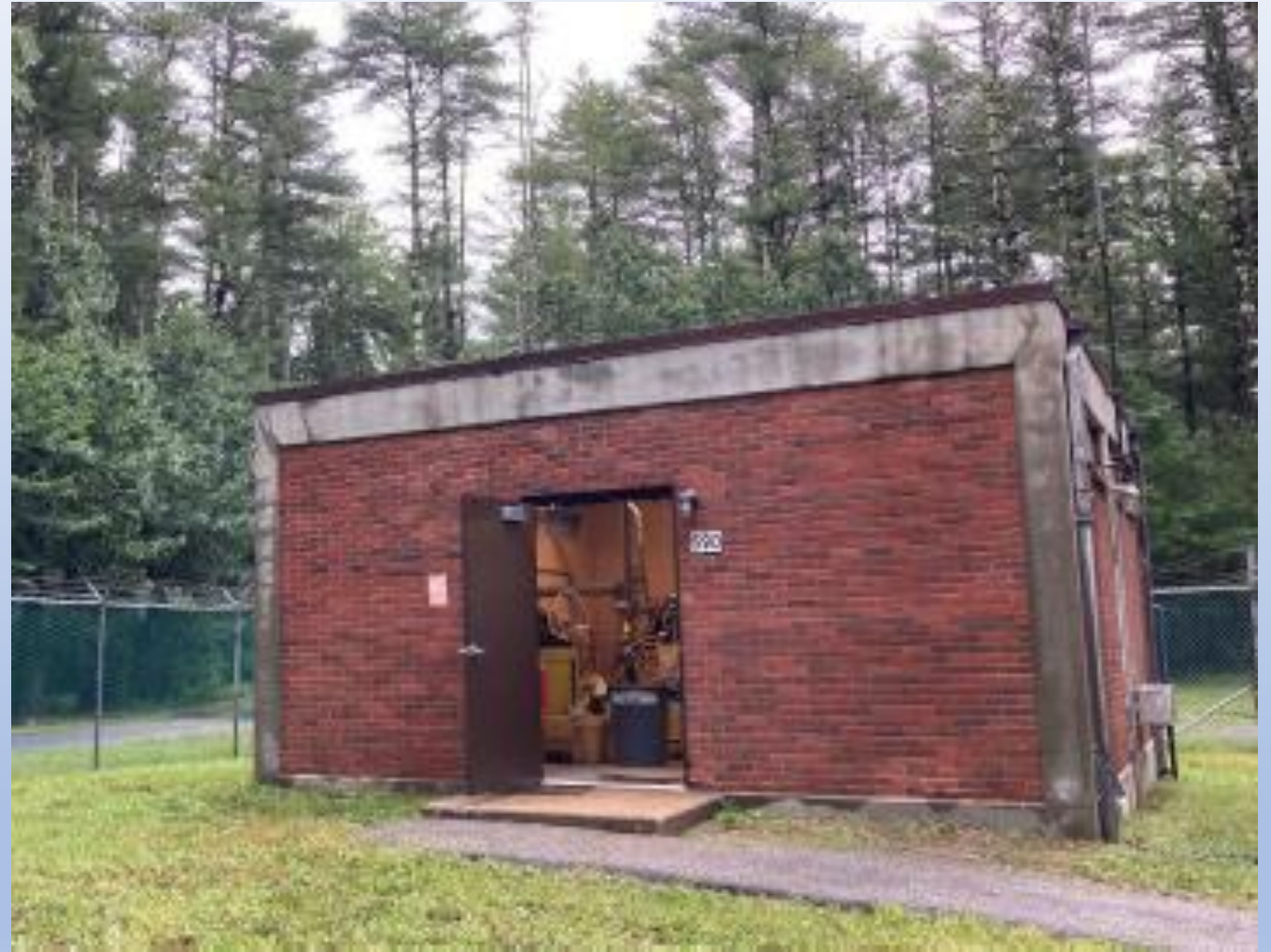
Mayflower Well No, 1 Pumping Station
