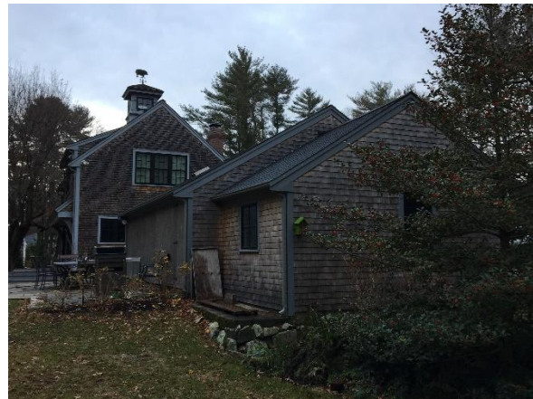
South w/Rear Addition
