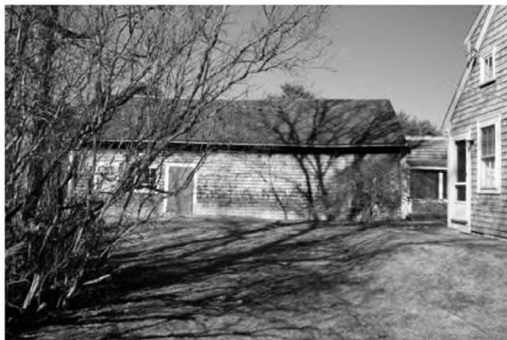
Connecting barn at NW of main house; south elevation.
