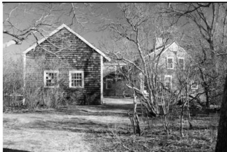
West elevations; connecting barn, rear ell, and main house.
