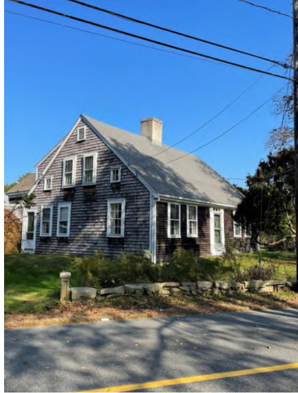
Close-up view from Temple St. looking East
