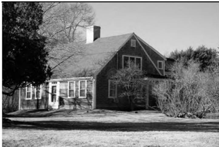
Façade and east elevation.
