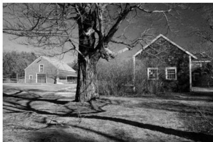
Free-standing barn and connecting barn; view from west.
