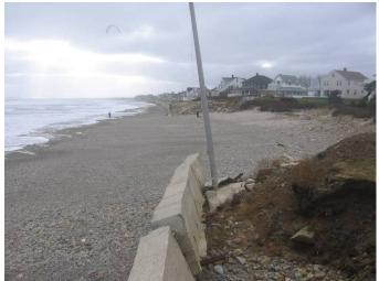
PHOTOGRAPH 35 - FAILURE OUTWARD ROTATION
