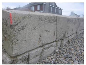
PHOTOGRAPH 36 - DETERIORATION OF CONCRETE
