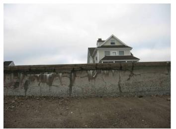
PHOTOGRAPH 41 - SIGNIFICANT CRACKING STA 203+00
