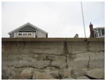
PHOTOGRAPH 55 - HEAVY CRACKING
