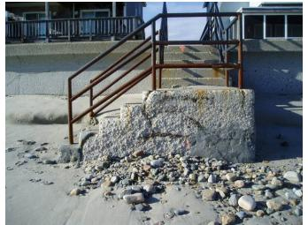
PHOTOGRAPH 4 - ABRASION, CRACKING AND PATCHING ON STAIRS AT 106+00
