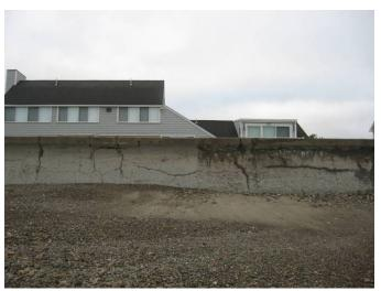
PHOTOGRAPH 40 - SIGNIFICANT CRACKING 202+00
