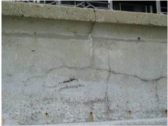
PHOTOGRAPH 53 - WALL TIES EXPOSED W/ STAINING AND CRACKING
