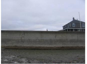
PHOTOGRAPH 18 - UNDERMINING FOUND ON 11/11/10 STA 122+00
