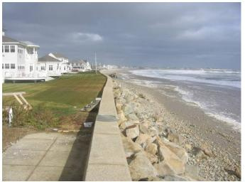
PHOTOGRAPH 17 - WALL CURVATURE AND DEAD GRASS BEHIND (OVER TOPPING)
