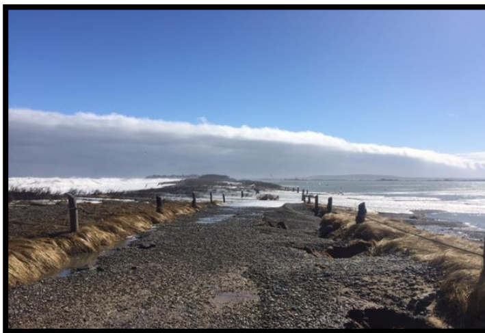
Significant coastal storm damage at Duxbury Beach after a blizzard in February 2014 (top 2 photos) and Winter Storm Riley, March 2018. Photo: Duxbury Beach Reservation, Inc. Facebook
