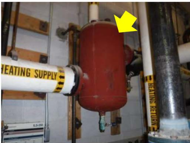
Tank Insulation – the air separator is not insulated which is leading to unnecessary distribution losses (Chandler ES).
