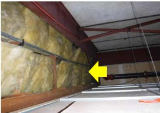
Buck Frame Sealing – the rough opening gap at the window between the wall and the window frame was not sealed above the drop ceiling; this gap is allowing air leakage around the window system (Chandler ES).
