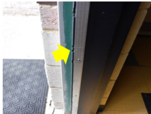
Door Weather Stripping – the existing weather stripping is damaged and is no longer stopping air infiltration/ exfiltration at the perimeter of the door system (Alden ES).
