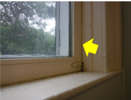
Double Hung Window Weatherization – the upper and lower sash of the window is partially painted shut; the gaps and cracks in the paint at the joints of the window and the casing are pathways for unwanted air leakage (Town Hall Old).
