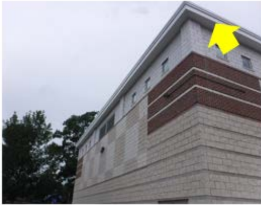
Roof-Wall Intersection Air Sealing – the exterior flashing and finishes at the roof-wall intersection are not constructed to stop air leakage (Alden ES).
