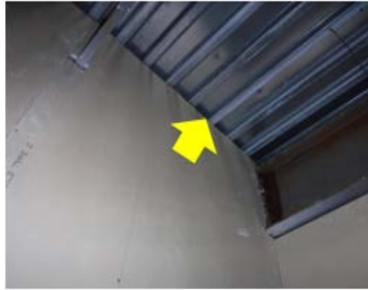
Roof-Wall Intersection Air Sealing – gaps between the roof deck and the wall framing are pathways for unwanted infiltration/ exfiltration (Alden ES).
