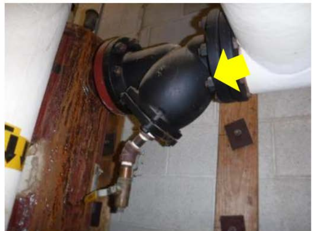
Valve & Fitting Insulation – the strainer is not insulated which is leading to unnecessary distribution losses (Chandler ES).
