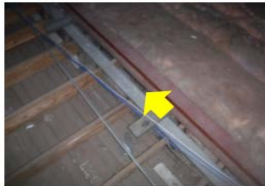
Attic Air Barrier Retrofit – there are gaps in the existing air barrier in place separating the unconditioned attic space from the conditioned office spaces. This allows for unwanted air leakage (Town Hall New).
