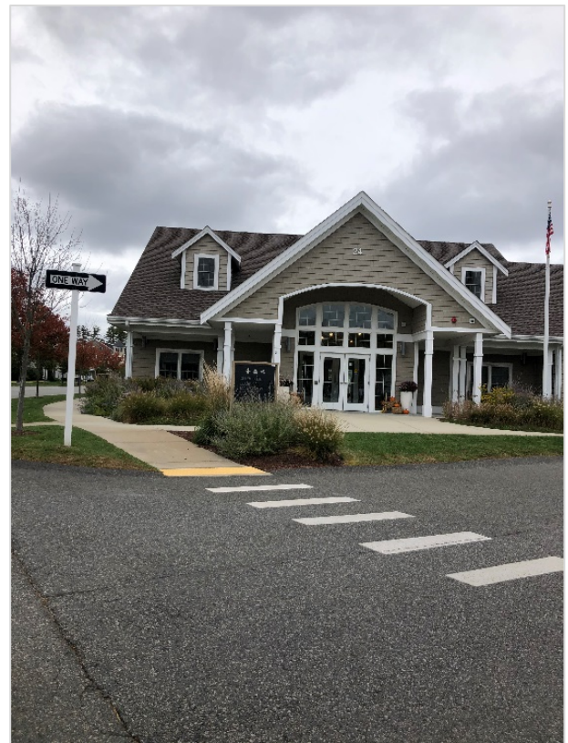
Compliant curb ramps should point users directly across the street to the receiving curb ramp and include tactile warning panels, as shown here across Tremont Place in Island Creek Village. Photo: HSH
